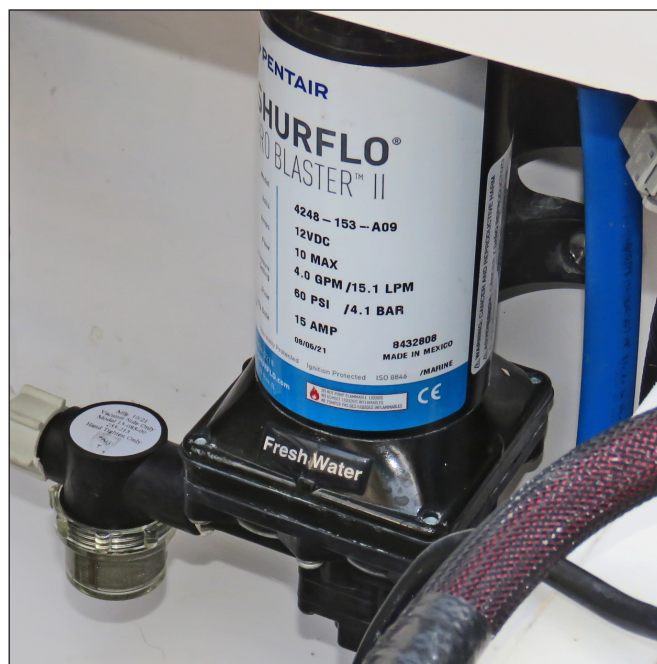
Fresh Water Pump & Strainer
