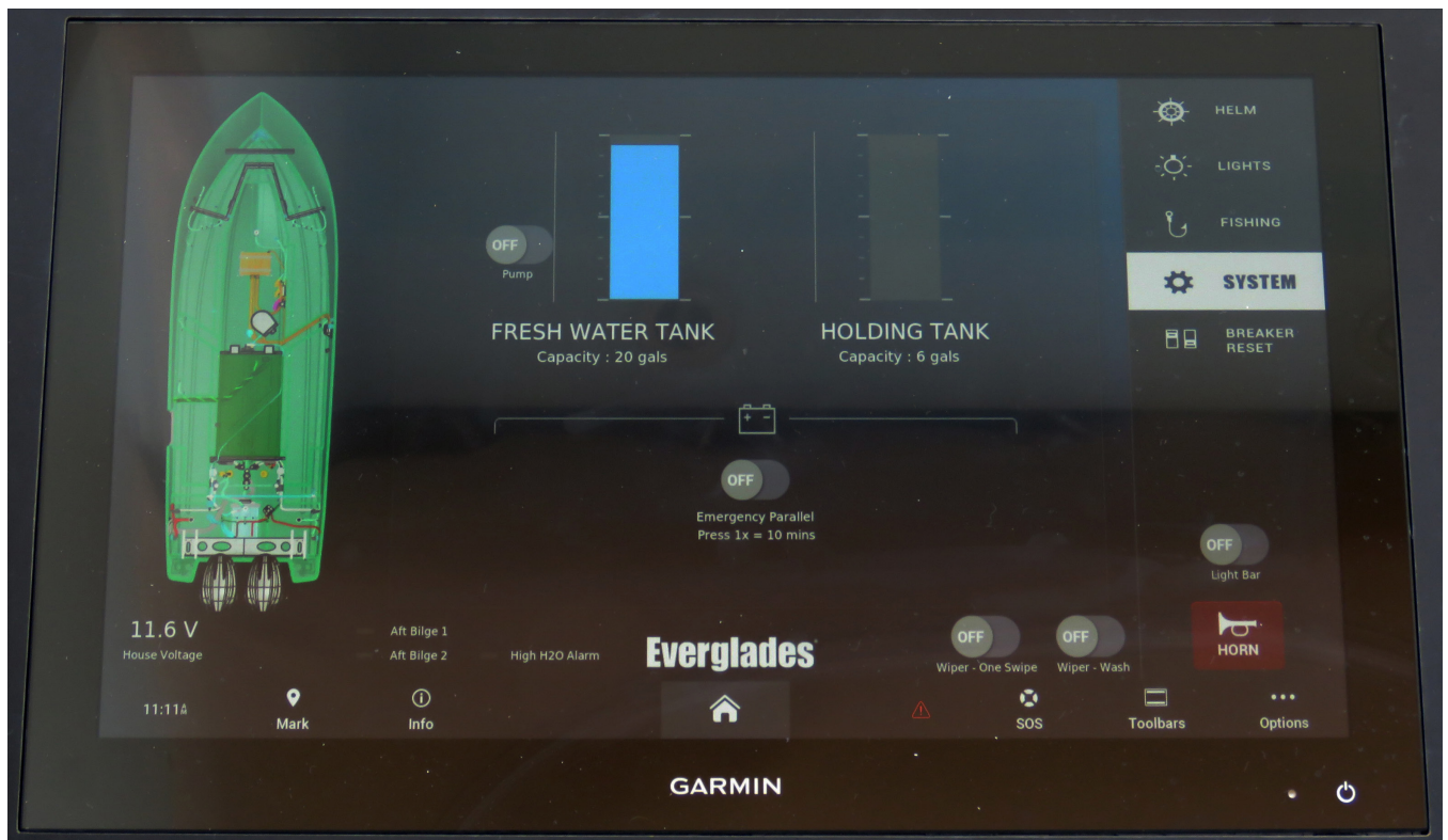
Typical Fluid Level Monitoring Screen
