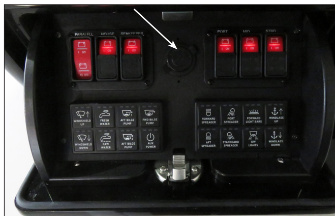
12 Volt Receptacle in Helm Switch Panel
