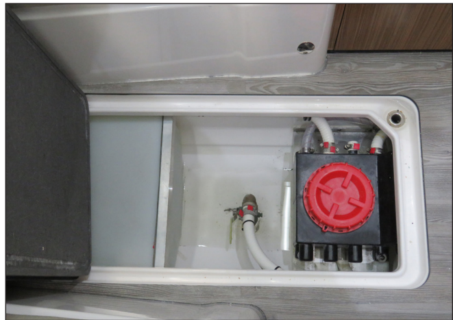
Removable Cabin Floor Panel & Cabin Drain Sump System
