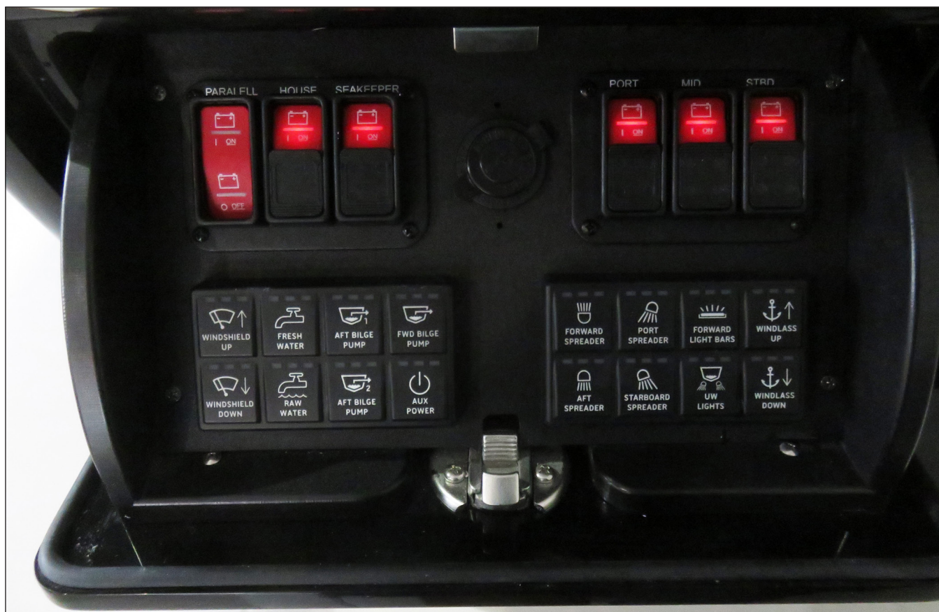
Port Helm Accessory Switch Panel & Battery Switches (Located in a lockable compartment on the port side of the helm)
