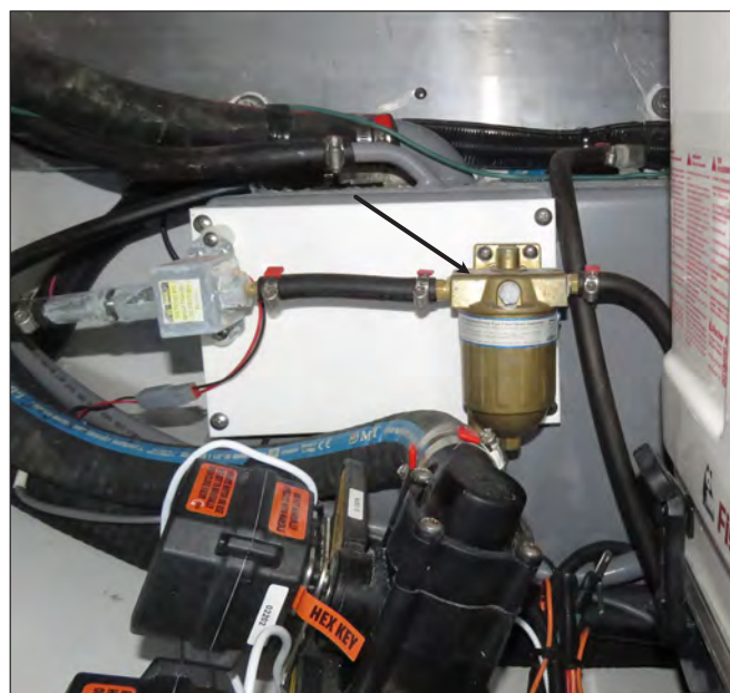
Generator Diesel Fuel Filter
