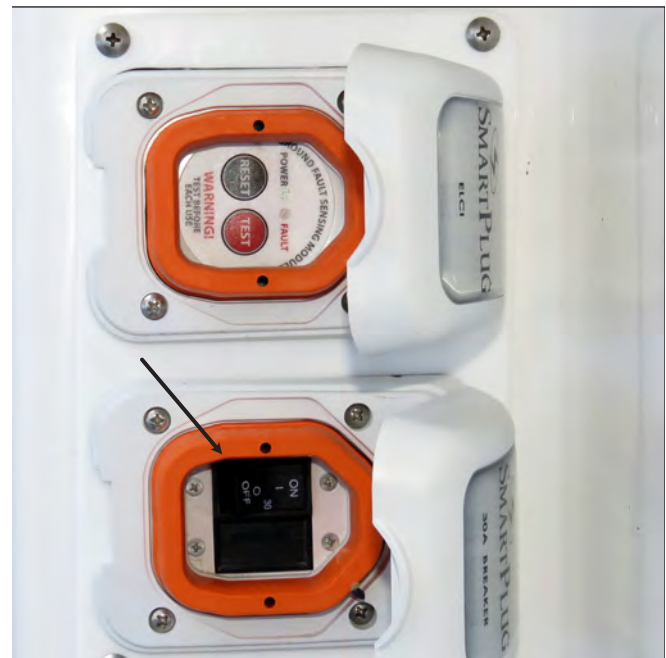
Inlet Main Circuit Breaker
