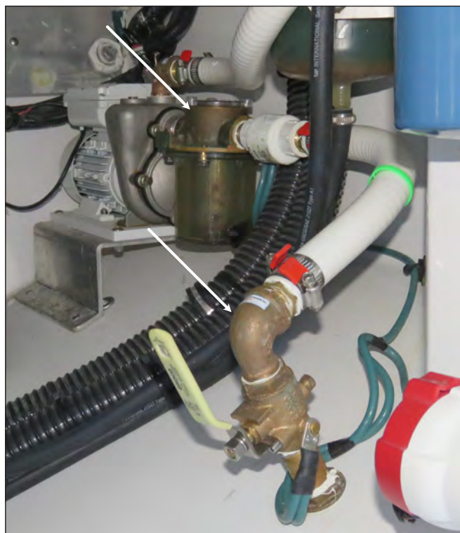
Air Conditioner Pump Strainer & Thru-Hull Valve
