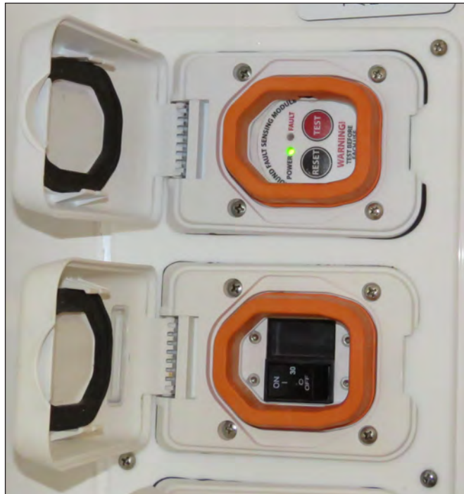
Typical ELCI Panel & Inlet Main Breaker
