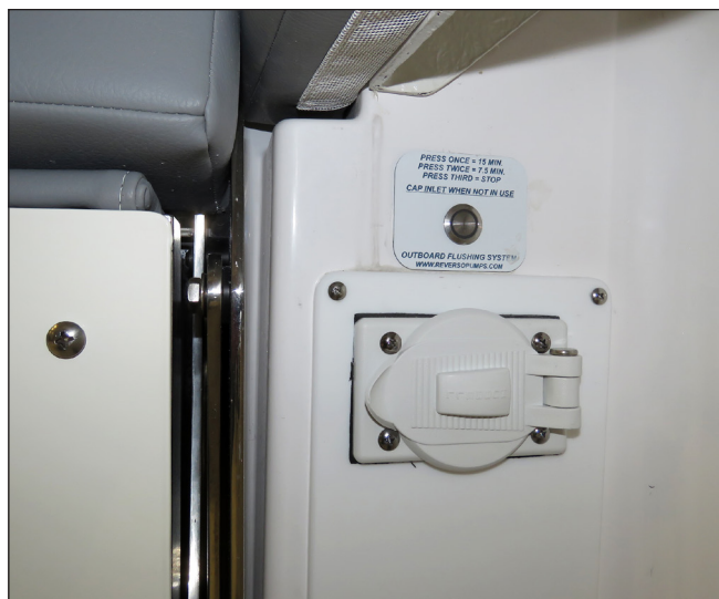
Aft Port Side Power Port & Engine Flush System Switch
