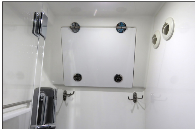
Upper Access Door in Shower
