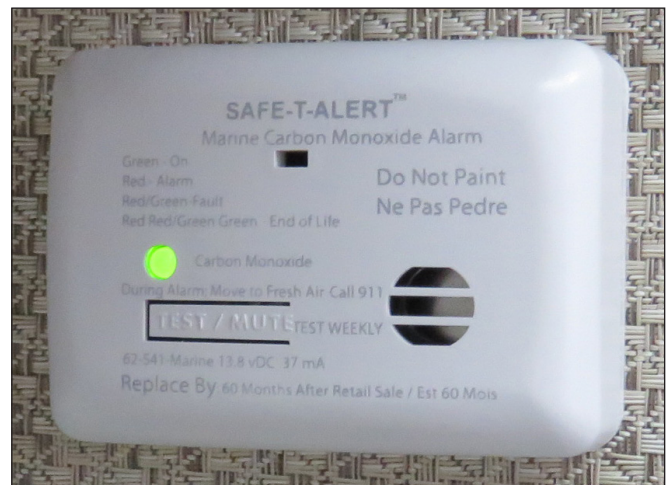
Cabin Carbon Monoxide Detector
