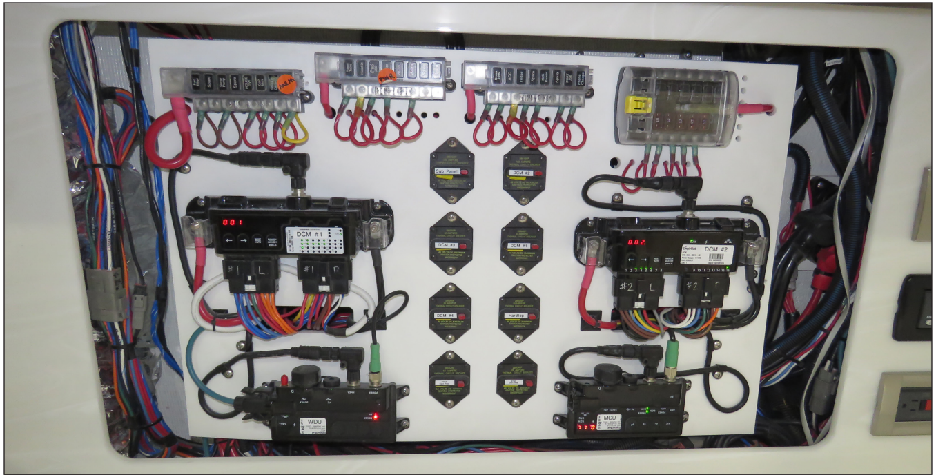
Digital Switch Control Modules & Main Circuit Breakers
