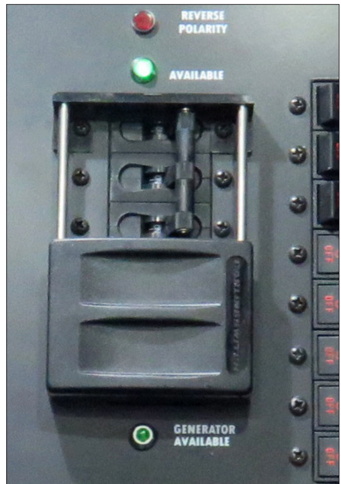
Reversed Polarity Light, Power Available Lights & Shore Power/Generator Main Breakers
