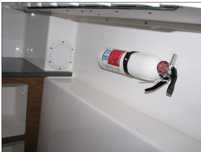
Fire Extinguisher on Forward Bulkhead
