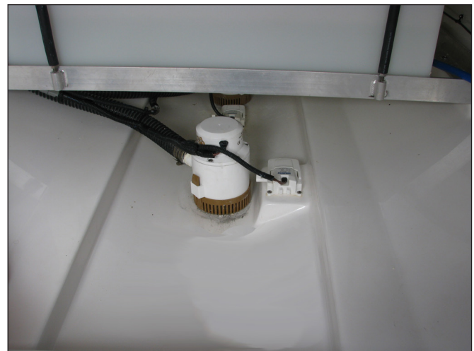
325 Center Console Aft Bilge Pump and Automatic Switch
