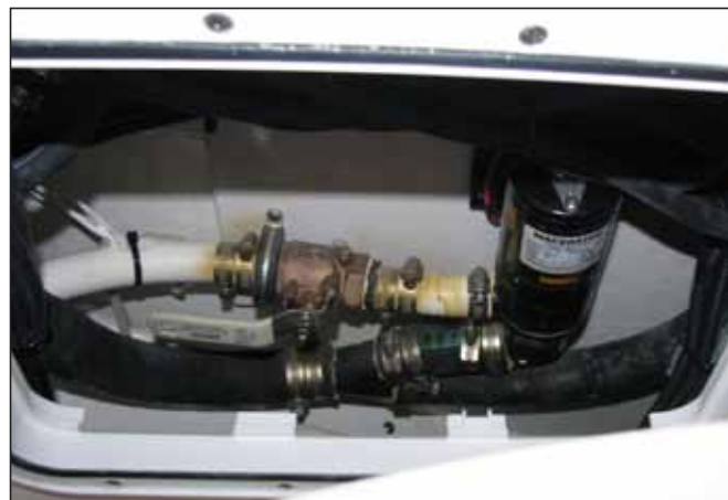
Macerator Pump and Discharge Valve
