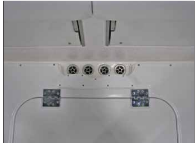
Typical Scupper Drains and Drain Rail
