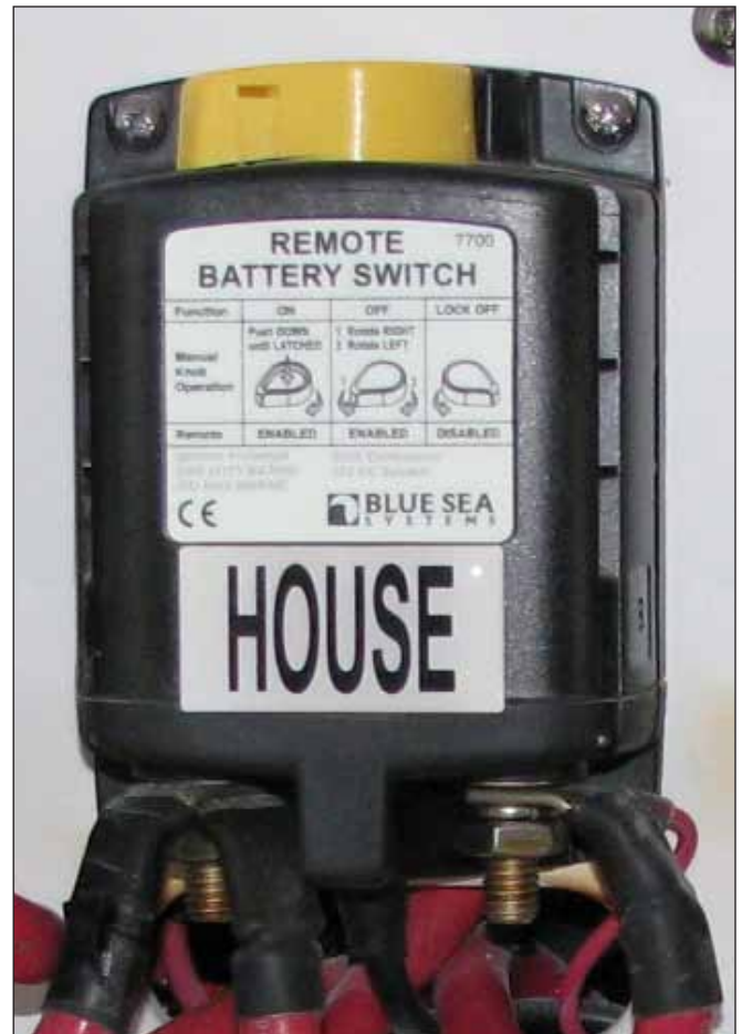
Typical Remote Battery Switch
