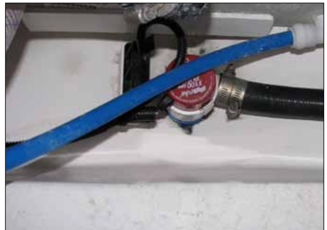
Aft Bilge Pump and Automatic Float Switch
