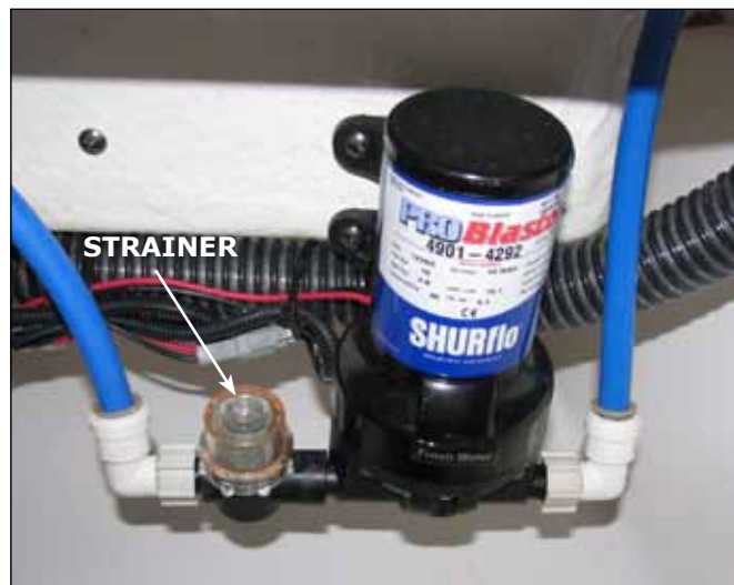
Typical Fresh Water Pump and Strainer
