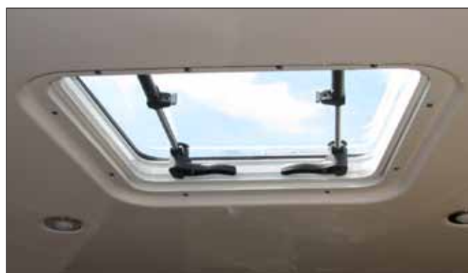
Deck Hatch Latched in the Vent Position
