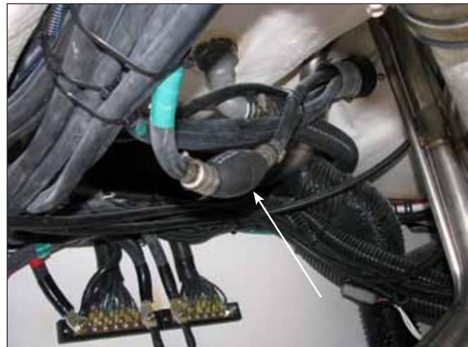
Primer Bulb at Rear Of Access Hatch
