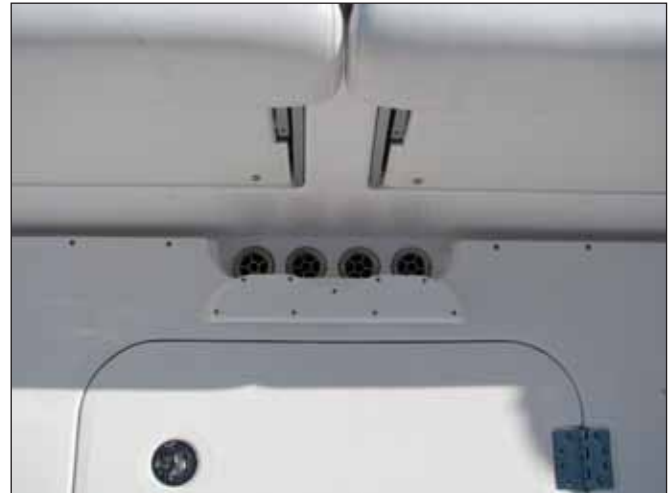
Typical Scupper Drains and Drain Rail
