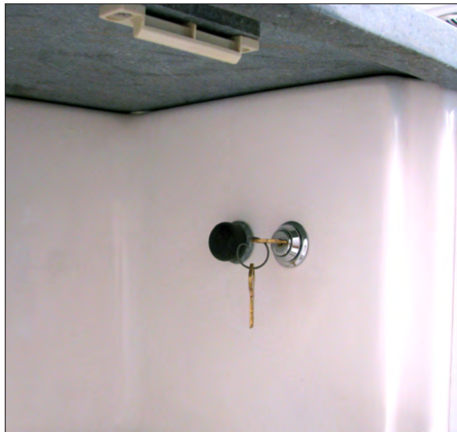
Typical Macerator Discharge and Key Lockout Switches In Compartment Near the Head
