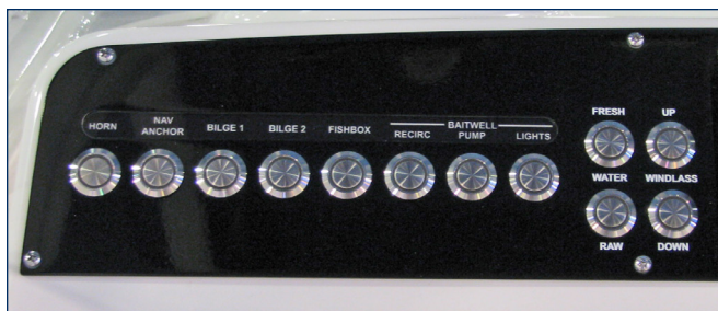
Port Side Helm Switches
