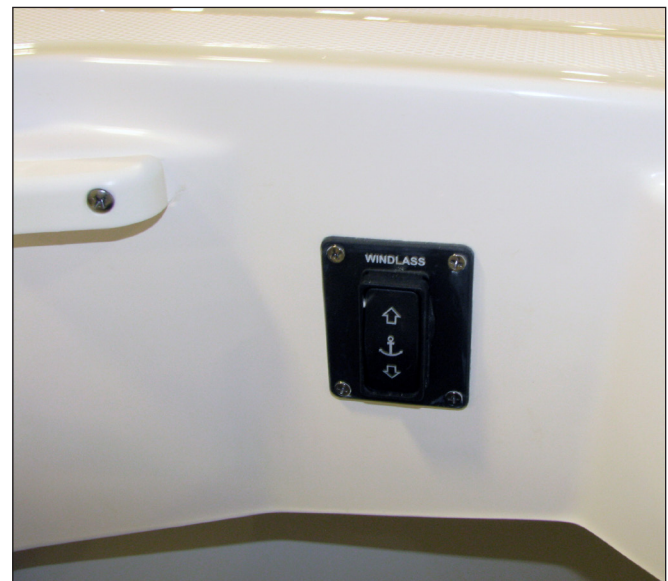
Anchor/Rope Locker Windlass Switch
