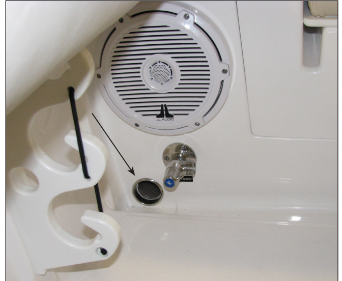
Cockpit Scupper Drain
