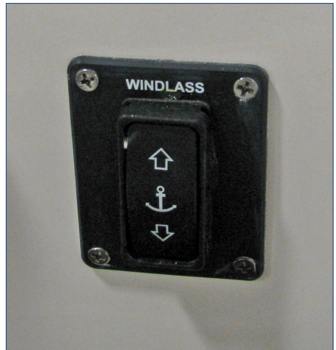
Anchor Locker Windlass Switch
